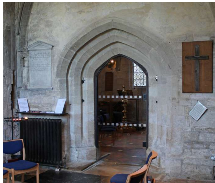
Frameless glass door to chapel – Burford Church
