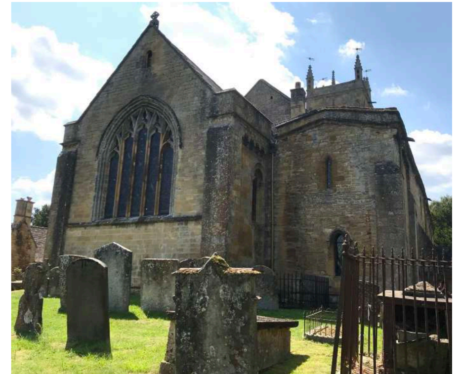
East Elevation of Chancel.
