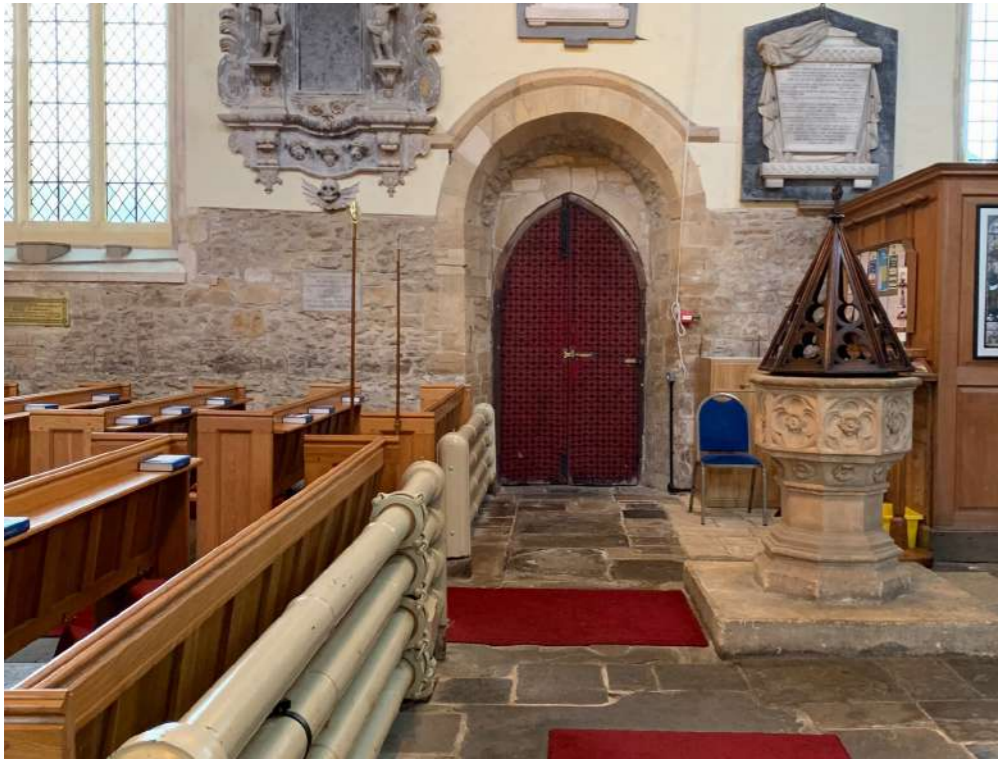
Font and South Porch doors.
