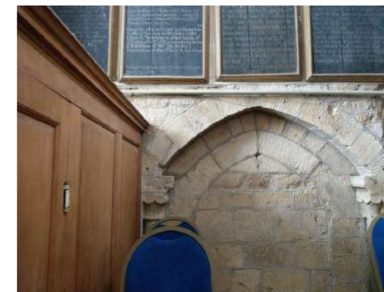
View from Nave showing blocked up entrance, inner arches and pointed arch bearing on Norman capitals and door jambs.
